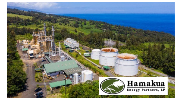
INDEPENDENT POWER COGENERATION
